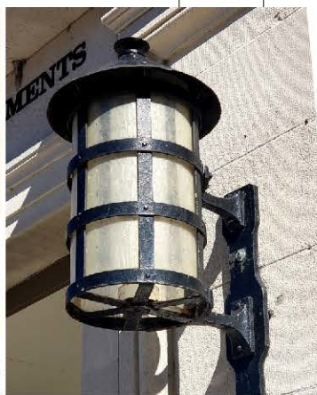
Choose fixtures that will focus light where it is needed; the sidewalk, people on the street, merchandise in windows, doors and gates. Reduce glare and light upward into residential windows.
