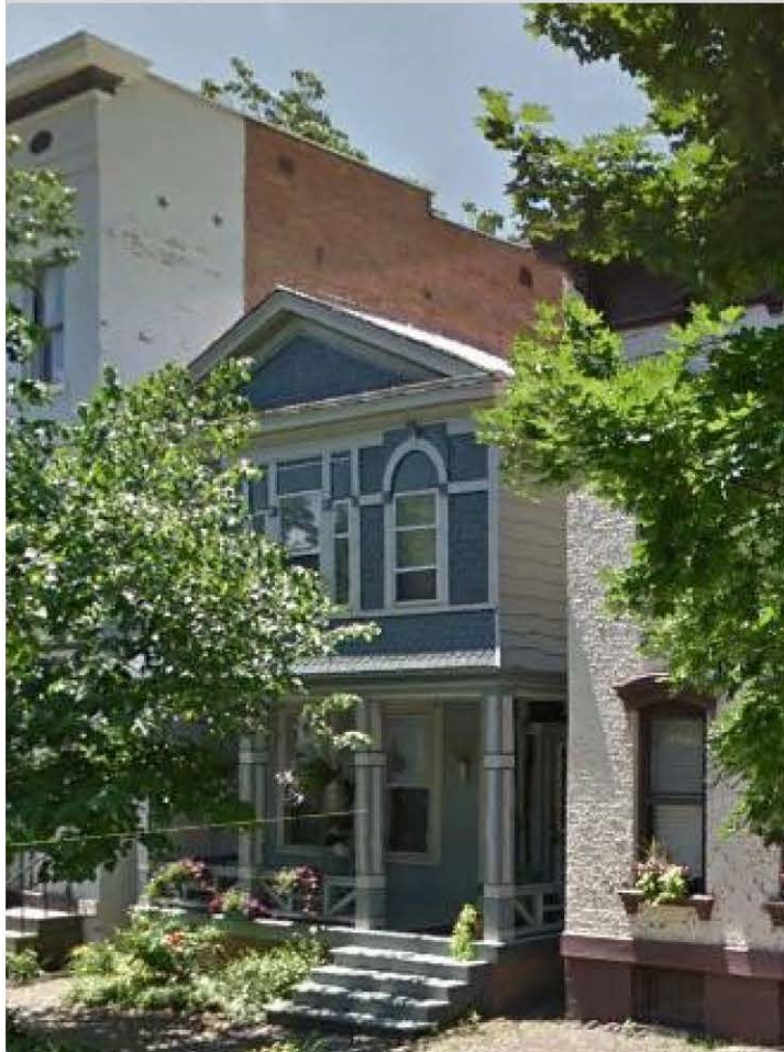
Porches are very rare in Troy's historic districts. So preserving their original features is especially important.
