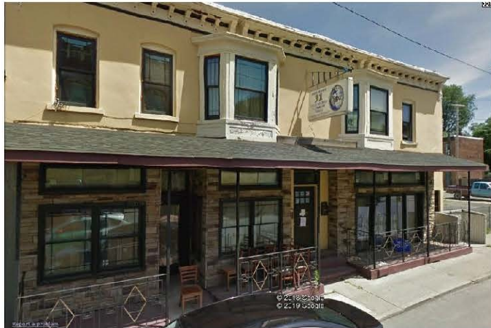
This inappropriate porch was added where none existed. The same effect could have been achieved for less expense with awnings and street furniture.
