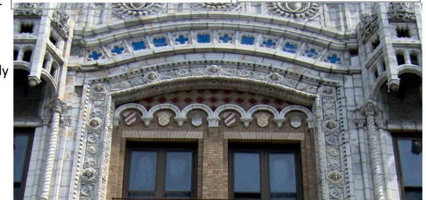
When masonry is clean, the detail is enhanced, and the craftsmanship can be fully appreciated.
