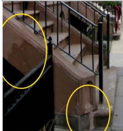
As with brick masonry, inappropriate sandstone patches are easy to spot
