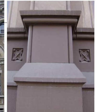
Cast Stone is a smooth concrete mix formed and pigmented to imitate the original stone.
