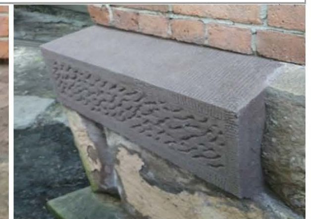
Stone building components that are beyond repair can be replaced with more durable materials, such as cast stone, glass fiber reinforced concrete and, in rare occasions, a resin component may be used.
