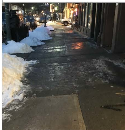
Don't allow building drainage to drip on a sidewalk and create dangerous icing.
