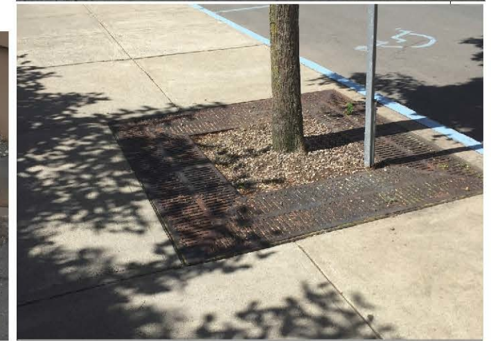
Tree grates must be no more than 1/2" out of level with the surrounding sidewalks.
