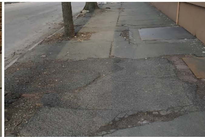
Asphalt, or macadam, is not allowed to be installed as a sidewalk surface.
