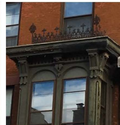
Cast iron cresting is rare now and should be preserved with a good coat of paint
