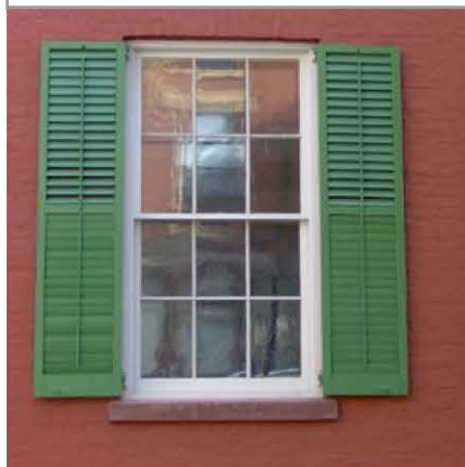
Above: shutters sized and installed inappropriately Below: wood shutters on hinges can cover the window
