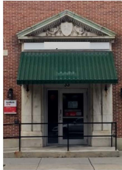
Contemporary metal awnings are not appropriate and this awning obscures the architec-
